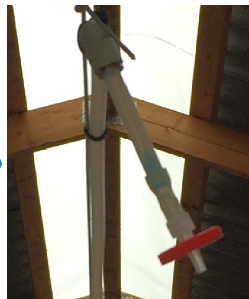
Figure 7b critical orifice and filter
