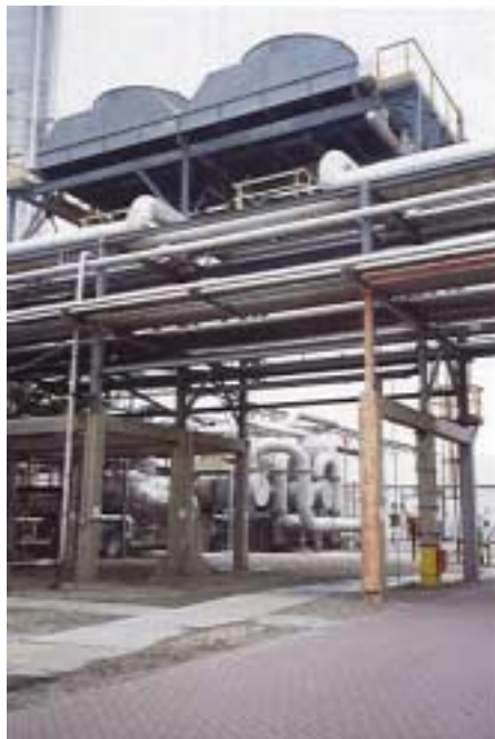
Figure 2.13: Example of a dry air-cooled liquid cooler in a chemical process [Pers. archive]
