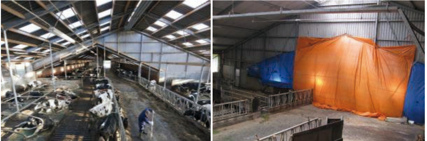
Figure 5: left, both barns are interconnected; right: the barns are isolated to avoid air exchange.
