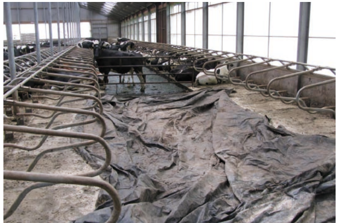
Figure 6: Closing cubicles and related floor area
