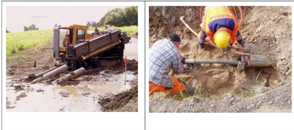
Figur 9 Etablering af underboring.
