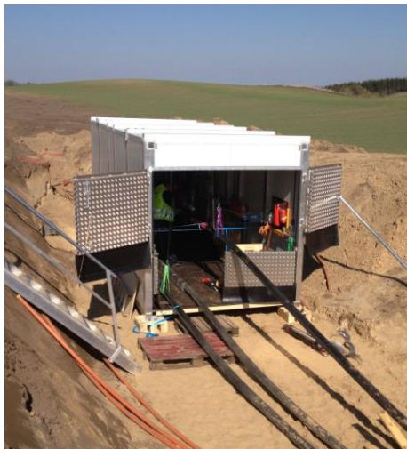
Figur 2-9 Montagecontainer placeret over en muffesamling
