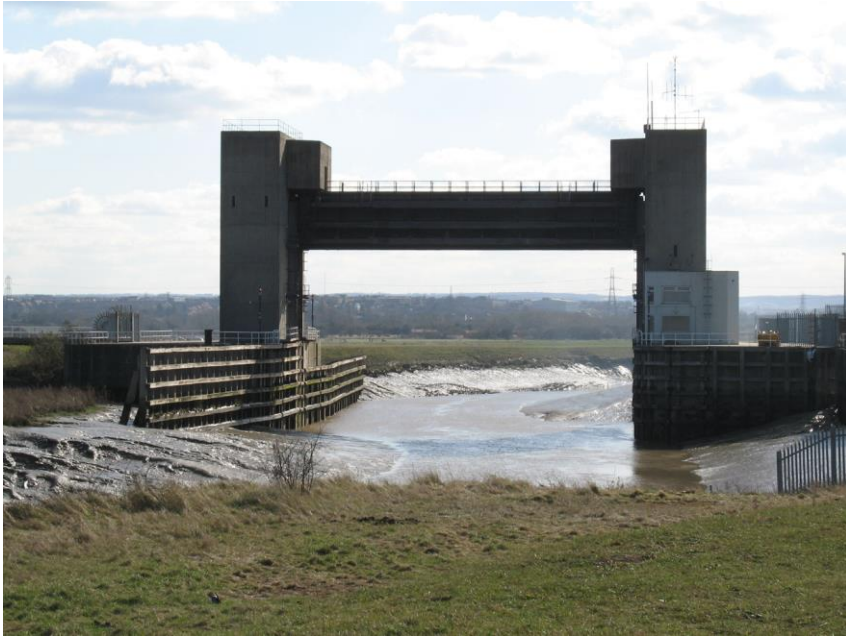
Dartford Creek Barrier
