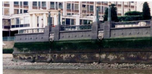
Concrete gravity walls
