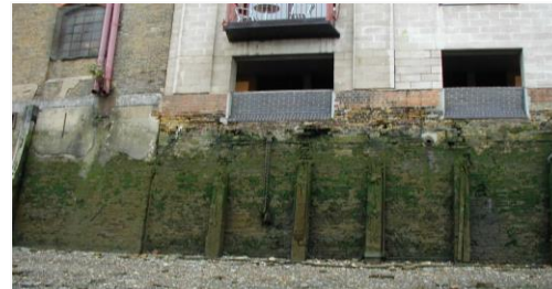
Masonry gravity walls
