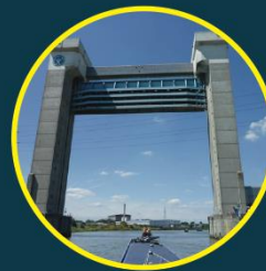
Barking Barrier (UK)
